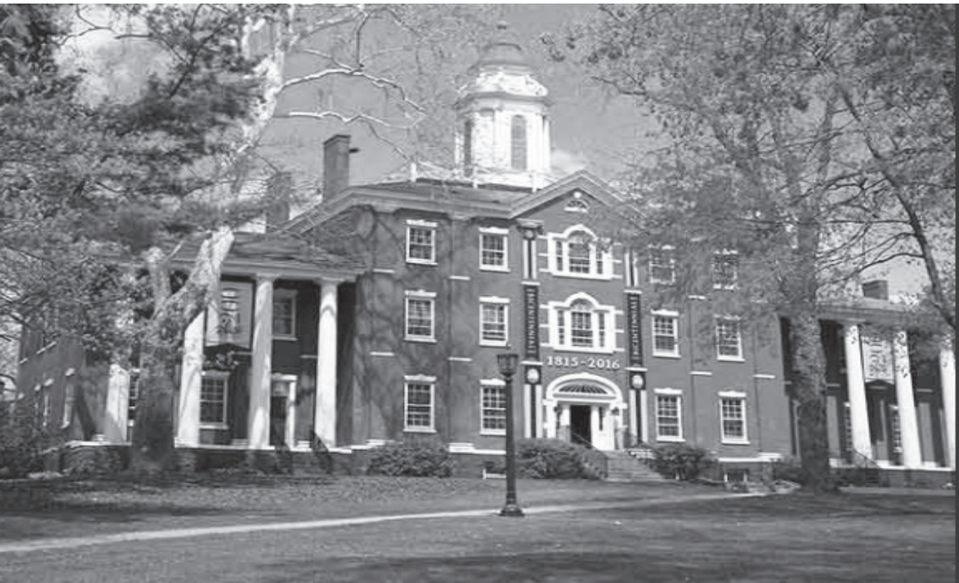
Bentley Hall in all of its glory prior to its Spring 2019 collapse.
