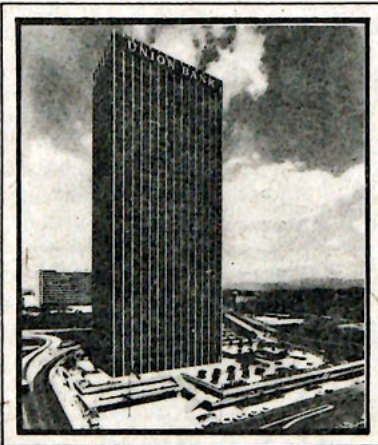
Union Bank Square, Los Angeles. One of several projects where Connecticut General dollars were put to work restoring existing cities.
