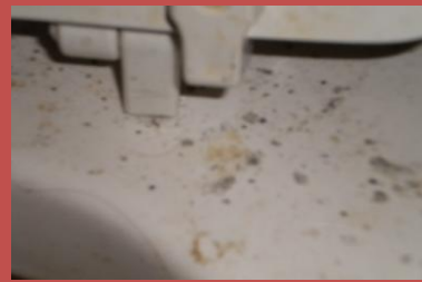
Figure Two: Mold on Toilet in House
