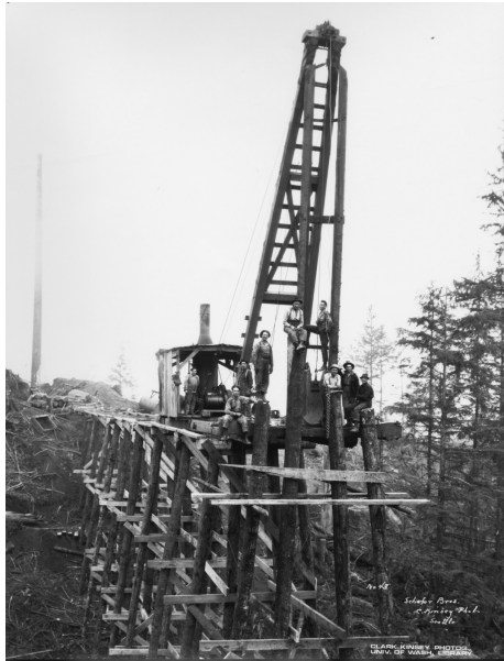
FIG. 8 Construction crew with pile driver on trestle under construction, Schafer Brothers Logging Company, probably in Grays Harbor County, Washington, by Clark Kinsey. c.1893–1945. Photograph. (Special Collections, University of Washington Libraries).
