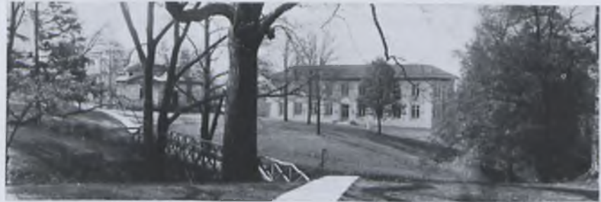
Looking across Ravine and Rustic Bridge toward Chemistry Building
