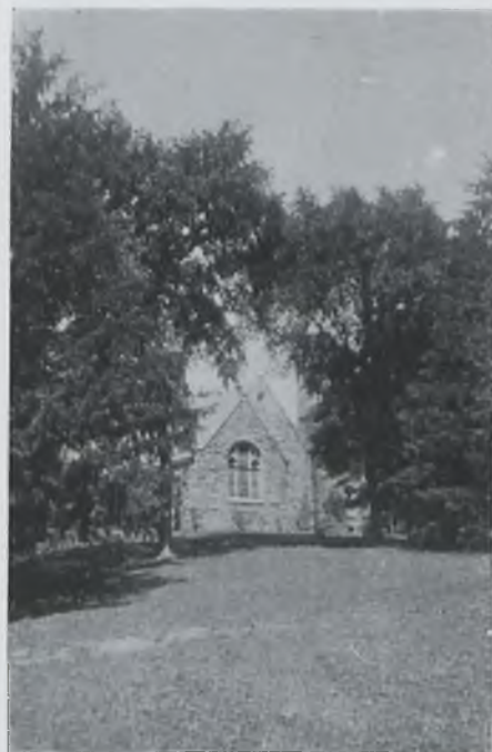
Ford Memorial Chapel, from the Rustic Bridge
