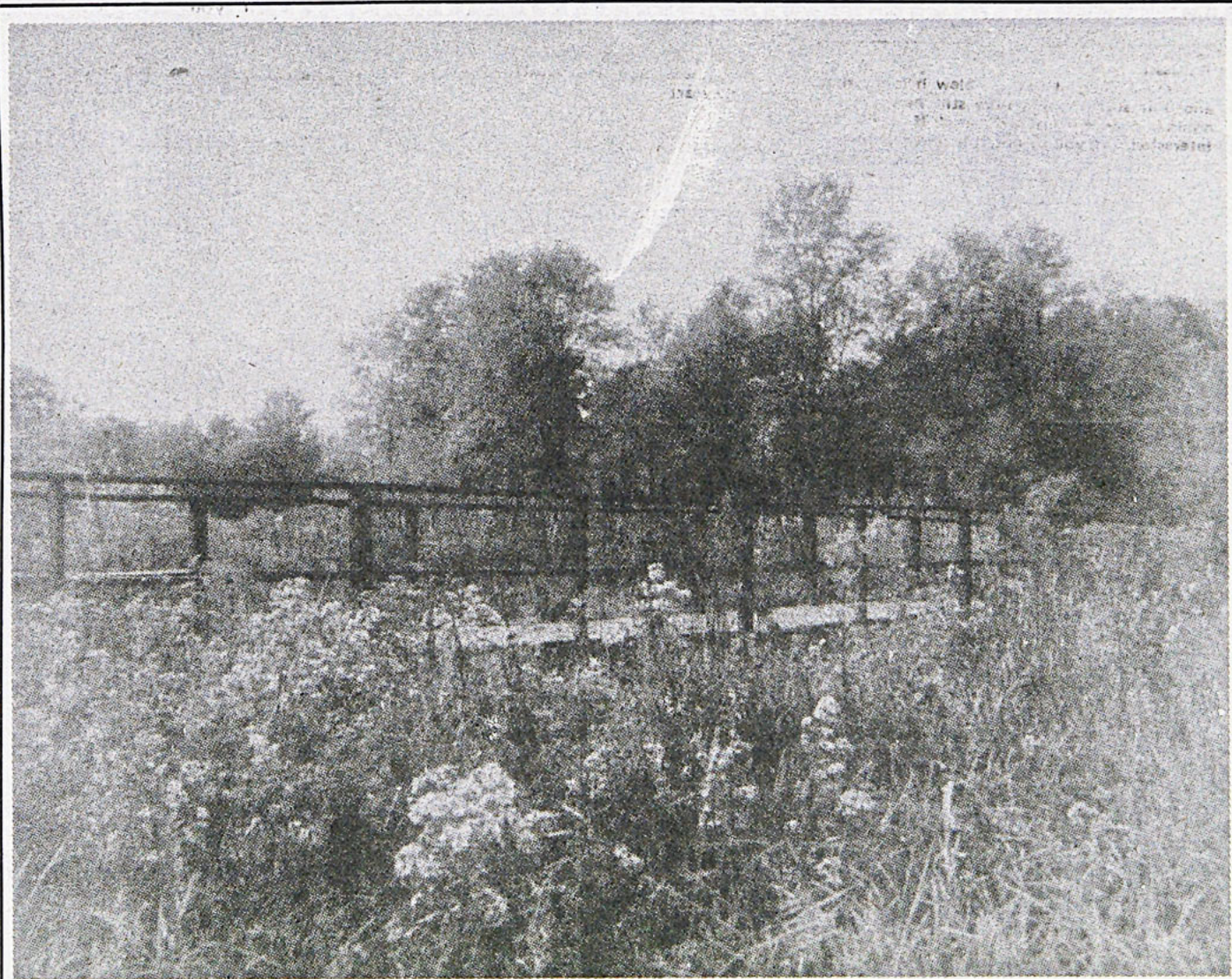
A small footbridge over wet marshlands.
