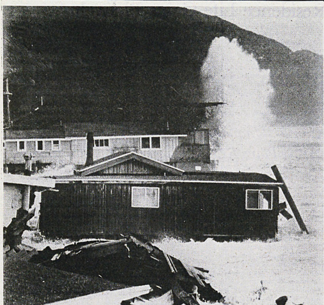
Waves up to 20-feet devastated the Calle section of Stinson Beach north of San Francisco during Tuesday's violent Pacific storm. At least three houses were destroyed by the waves and 18 others were severely damaged, a fire department spokesman said. AP Laserphoto
