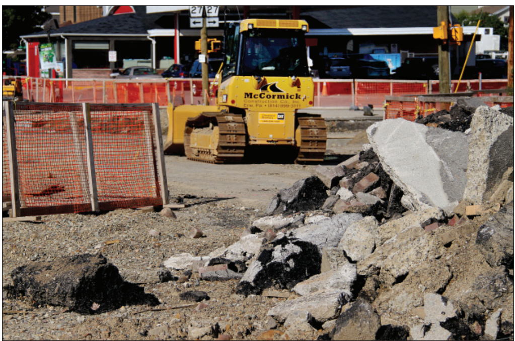
MEGHAN HAYMAN/THE CAMPUS Road crews leave the N. Main Street and North Street intersection site at a standstill as they take a break from construction.
