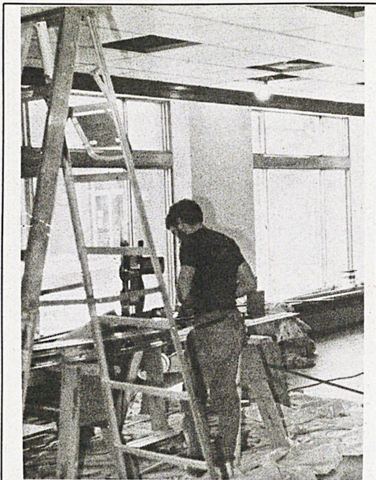
A construction worker saws as renovation continues in the Admissions Office.
