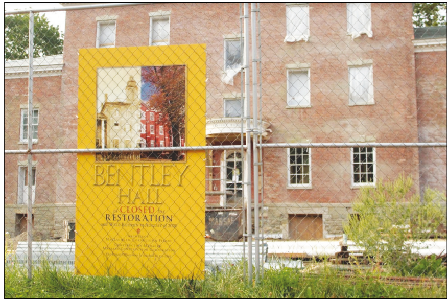
Top Left: Notice outside Bentley Hall advertising its closure due to renovations. Construction work outside of historic Bentley Hall as it nears its completed renovation date.
