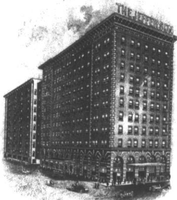
HOTEL JEFFERSON AND ANNEX BOTH FIRE-PROOF JEFFERSON AND LIBERTY
